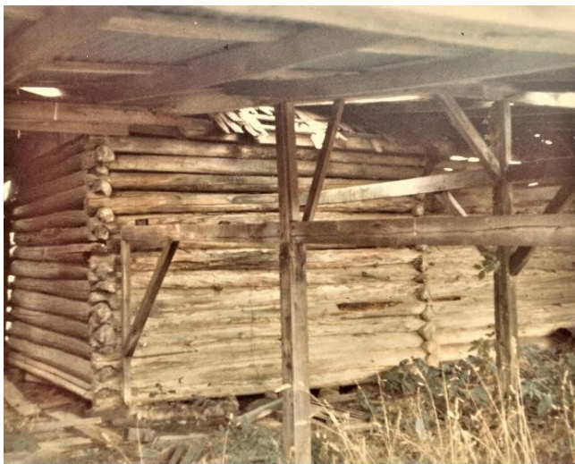
Figure 12: Photographer unknown, before Fall 1974. Reproduced from Reed 2023, Image 16.
