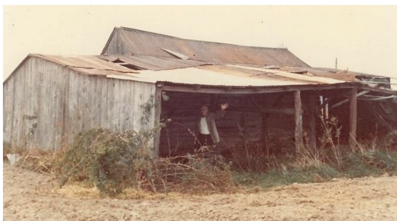
Figure 7: The log stable with rear open shed addition supported by posts. Unknown photographer and date. Same man as in Figure 6. Image courtesy of CCHS. Reproduced from Reed 2023, Image 14.
